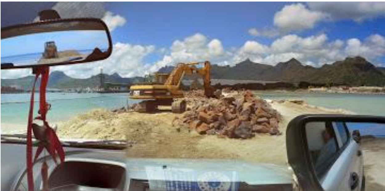
ROCK REVETMENT AND COASTAL PROTECTION WORK AT FORT WILLIAM AND FORT GEORGE MAUTITIUS PORT AUTHORITY
