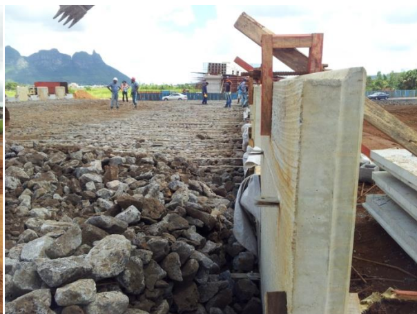
OUR TEAM ARE PREPARING THE BLINGDING AND ALIGNMENT FOR PRECAST PANEL
