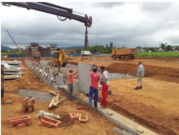
OUR TEAM ARE PREPARING THE BLINGDING AND ALIGNMENT FOR PRECAST PANEL
